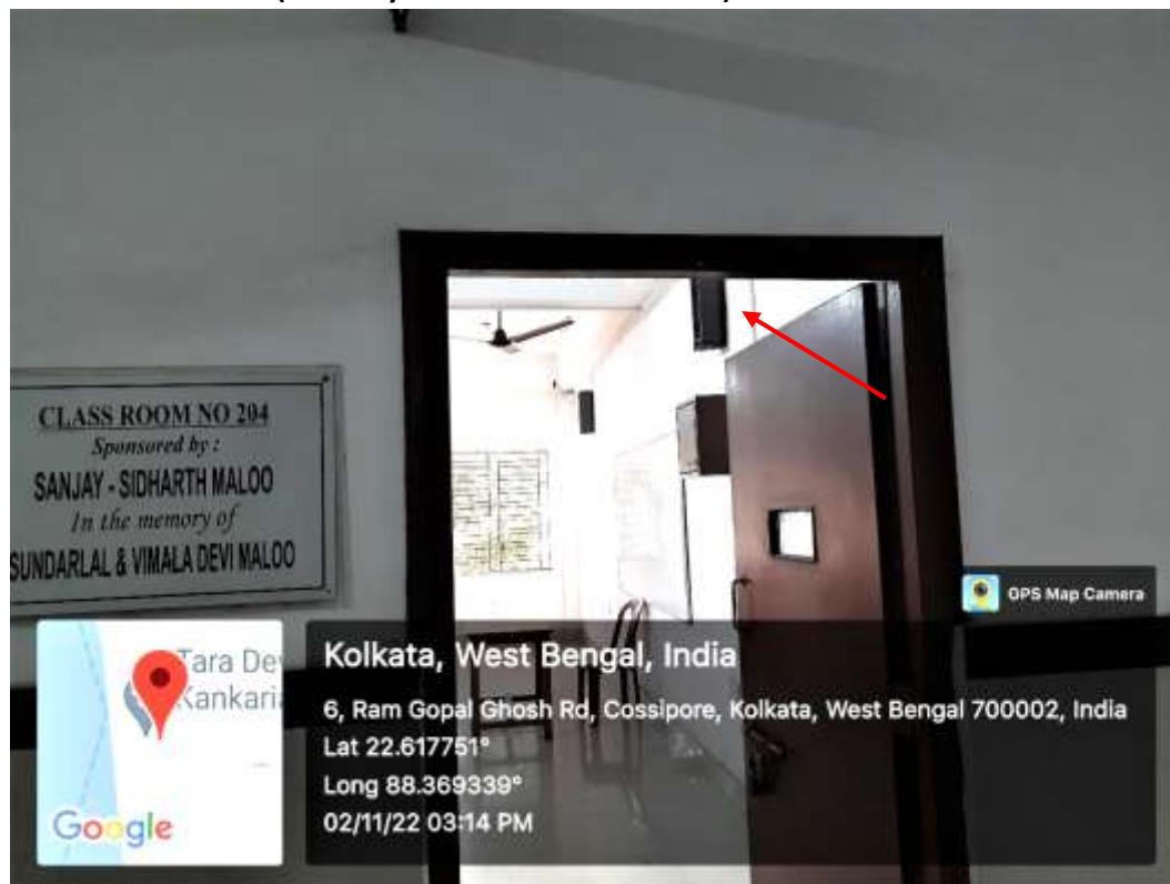
15. Classroom #204 (Audio system shown with arrow)
